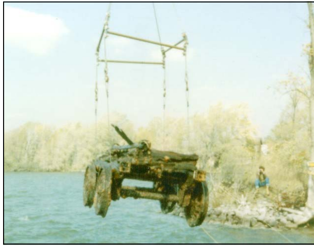
Above: In 1980 an original 1867 CP&MR&MCo Crossen built ore car was extracted from the Trent River. This is the only image of a Crossen car known to the author and this reveals little of its construction beyond the fact that it had four wheels. Parks Canada somewhere in one of its warehouses has stored this car since its elevation to dry land.
