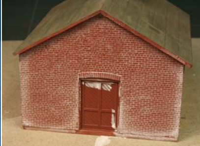
BRICK WALL PHOTO 2
