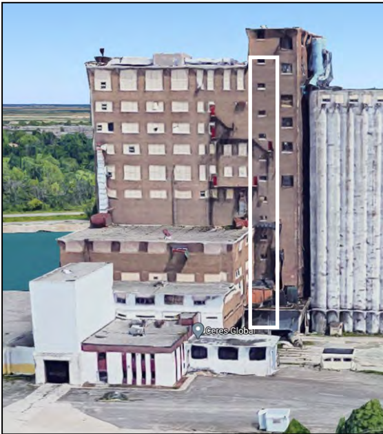
PHOTO 8 ABOVE: An enlargement of a Google Globe View image (a 3D graphical rendering from the 2D satellite image) made it possible to count the floors (white highlighted windows) in the brick milling structure alongside the silos.
