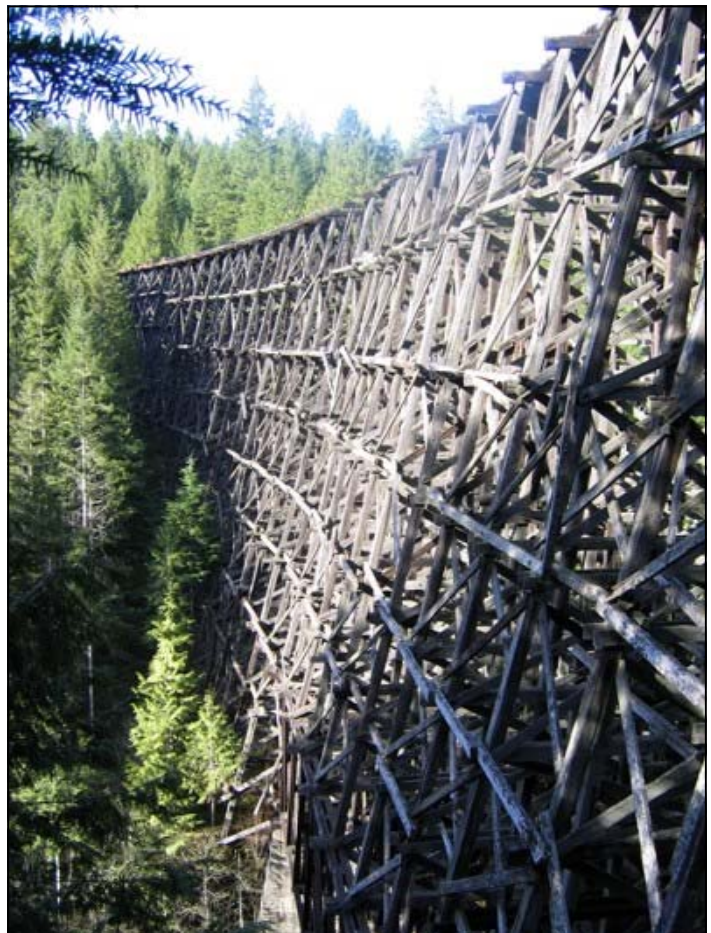
Right and Below: The Kinsol trestle is accessible by a short trail at the north end of Shawnigan Lake. It was the largest wooden trestle on Vancouver Island and carried CNR traffic from Victoria northwards until the late 1980's.
