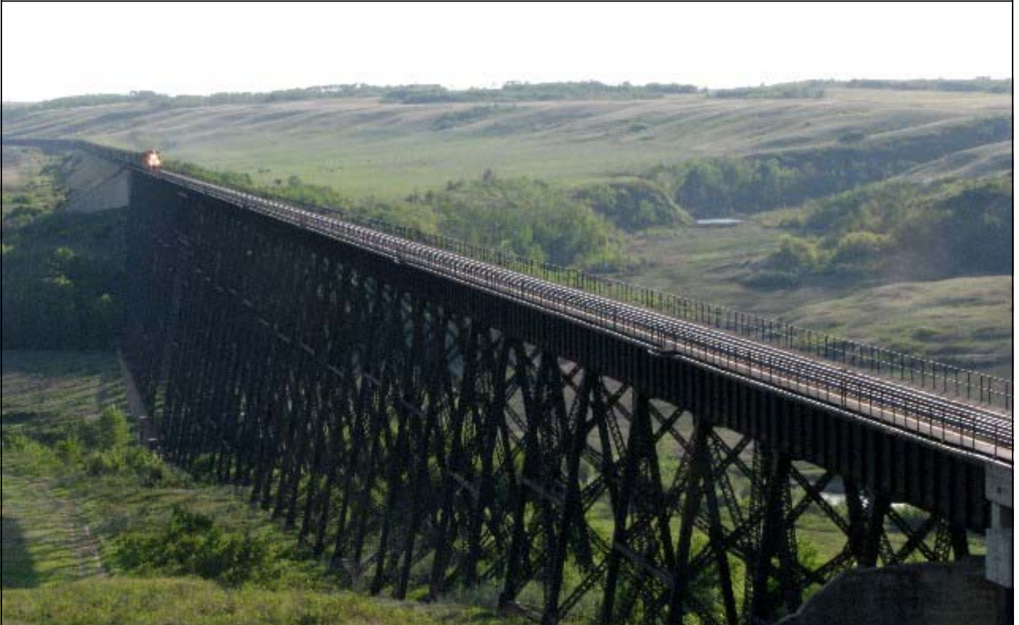
Photo Below: The impressive Battle River Bridge at Fabyan, AB, near Wainwright, AB, is a magnet for any serious railfan. Rolling onto the west end of the CN viaduct are units 2658 and 5862 with an eastbound train of hopper cars loaded with coal. Out of sight in mid train is a DPU. The Battle River has scarred the landscape with a deep gorge in the landscape that the Grand Trunk Pacific crossed with this marvellous example of bridge technology.
