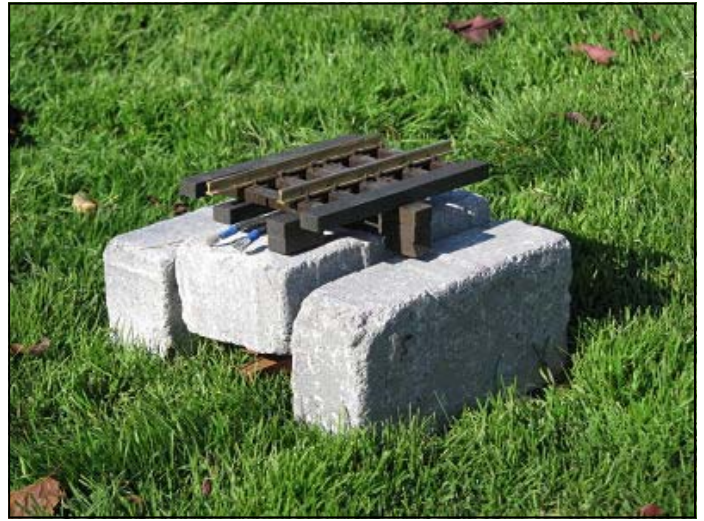
Photo Above: The components in place. The paving stones create the base of the roadbed. Two pavers line each side of the central paver. All stones are laid in earth in the manner illustrated with the two outside pavers below the top surface of the centre paver. On top of the central paver is one of George's track holders built up of cedar strips and painted black to represent creosote. Note the stacked cedar strips that descend the side of the central stone. A similar drop is located on the opposite side. These drops prevent lateral movement of the track holder. The track holder has a channel which acts as a holder to contain the electrical wires that lead to the turnout motors.
