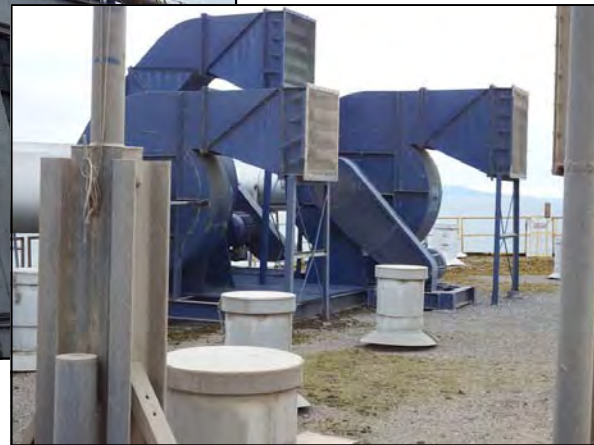
Photo Below: Walter Reid photo: Large exhaust fans are installed on the roof of the grain elevator to remove grain dust.
