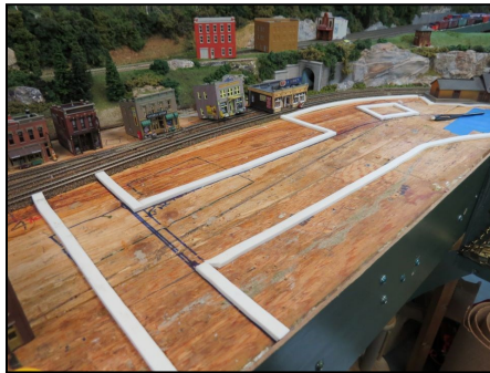
The roads in Nathansville have been "taped" out and are waiting for grout.
