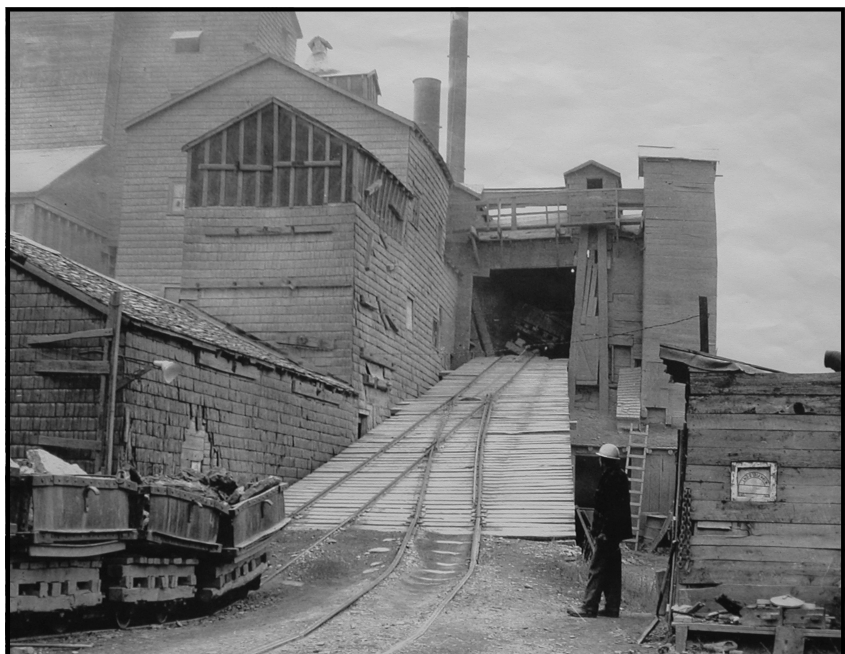
Photo 2: The prototype Kirkfield Crushed Stone Company as it was in 1961. Dump cars are pulled up the ramp into the crusher by a cable between the rails. Empty cars are returned through the spring switch to the receiving track on the right where they wait to be returned for loading in the quarry.
