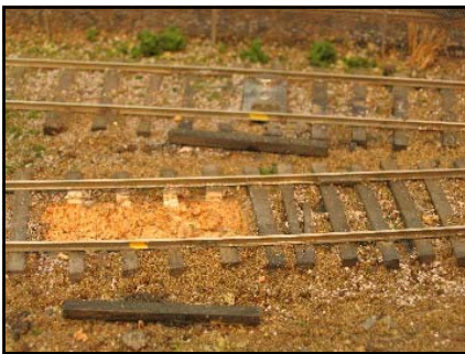
Photo 1: When installing a Kadee magnet a major excavation of track and roadbed is required.
