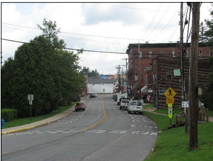
Photo above: Main Street Mount Jewett, Pa. Town runs at 45 degrees to track.
