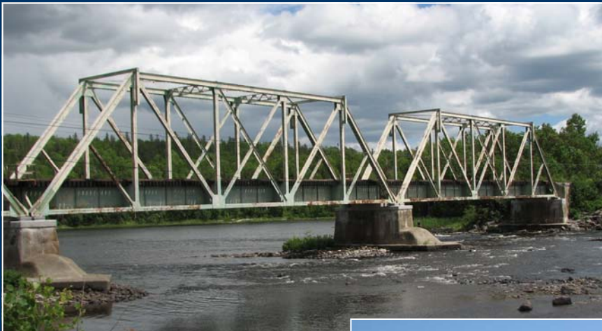
MONTREAL RIVER BRIDGE Latchford, Ontario
