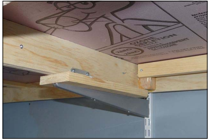
PHOTO 4 ABOVE: Shelf bracket detail
