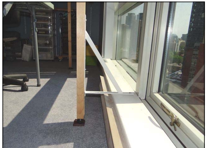
PHOTO 17 BELOW: Legs of the bridged braced to the wooden sill.
