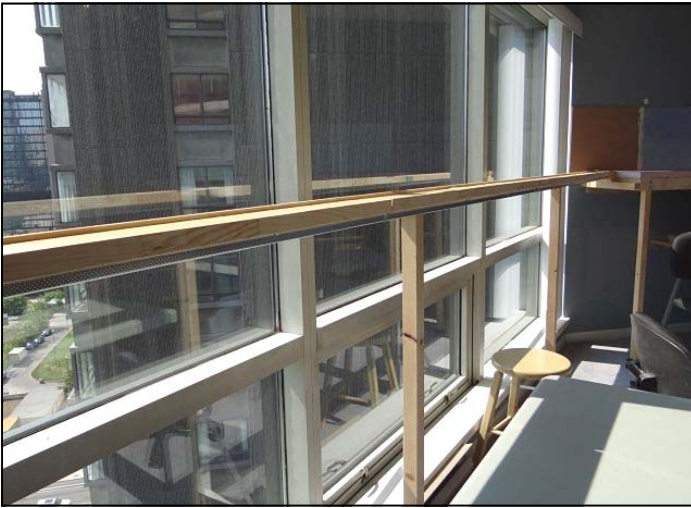
PHOTO 18 ABOVE: The finished 4m bridge.
