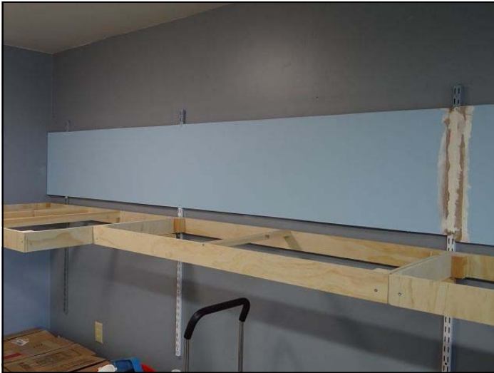
PHOTO 9 BELOW: The peninsula frame: construction detail.
