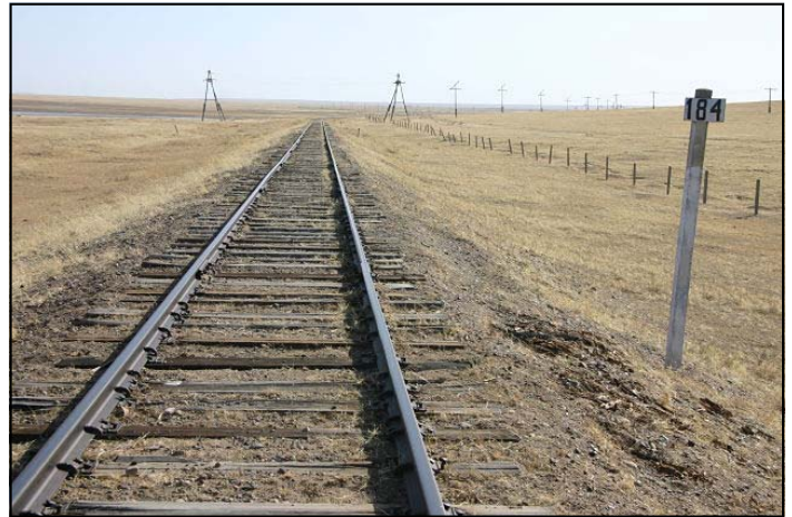
PHOTO ABOVE: Example of track laid directly on ground with only minor heaping of inorganic soil to provide drainage. Photo by the writer of the Russian gauge, Dornod branchline in Mongolia.
