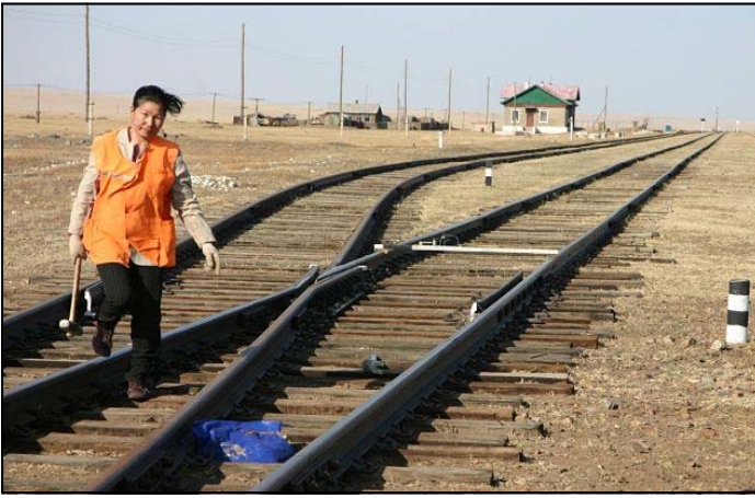
PHOTO 2 ABOVE: Same Dornod branchline as in photo 1, showing lack of track camber at siding and natural gravel beside switch ties. There are only three trains a week so the track worker can take her time.
