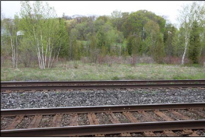
PHOTO 5 ABOVE: CN mainline double tracks at Port Hope with north track ballast replaced and south track still with older ballast.
