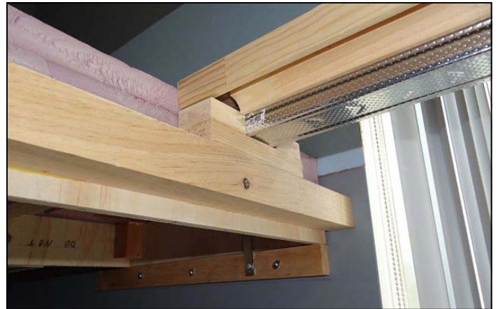
PHOTO 15 ABOVE: The wooden structure which will support the rails on the bridge (inverted). The steel girder will fit into the central channel (black clamp)
