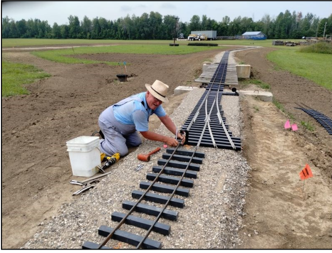
PHOTO RIGHT BY JOHN PARK: Subgrade finalized.
