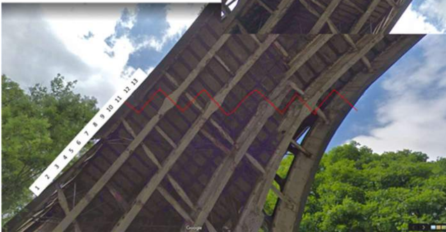
Approx. 13 cross beams on the centre span
